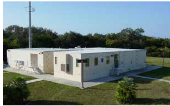
Draper designed and built the GPS Telecommunications Simulator Test Station at Cape Canaveral Space Force Station, Fla. The facility supports end-to-end system requirement verification and testing of satellites and ground system technologies.
